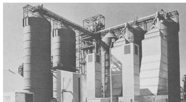
Twin towers at left can dry 15,000 tons of seeds daily.
